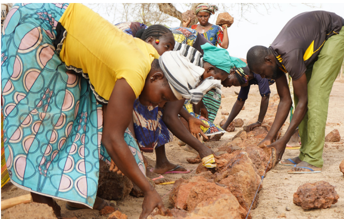
Women laying the stone barrier
